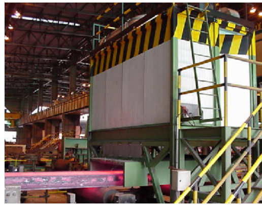
Fig. 10 - System installed in the continuous casting strand
