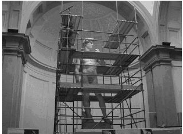
Figure 3b – The set-up installed for the measurement.
